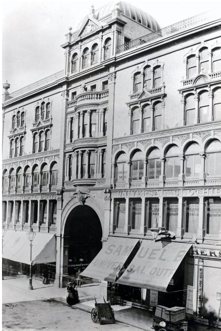
St Mary Street Entrance circa 1895 and 1975
